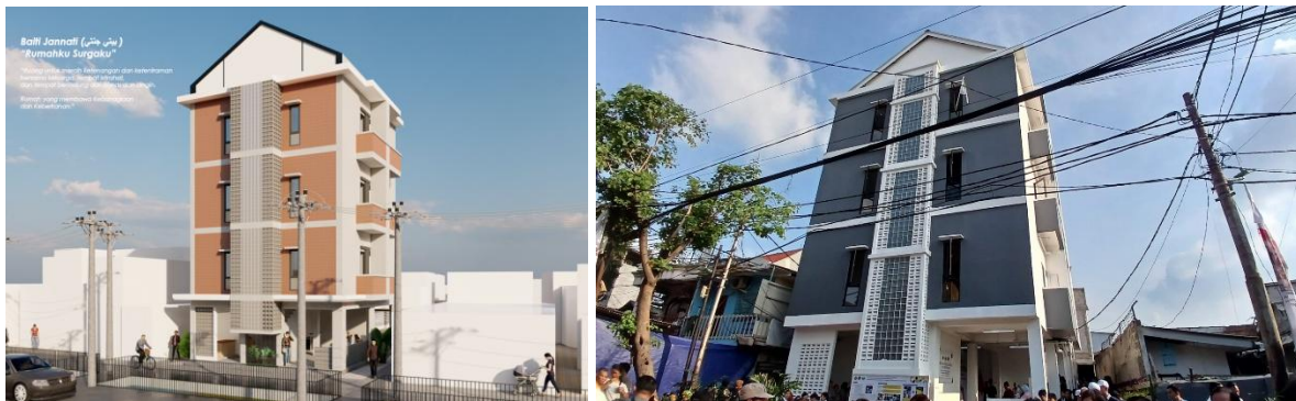
Figure 7. 3D Illustration and Final Construction Outcome
