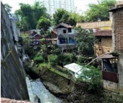
Figure 8. Cidadap river, between Hegarmanah and Ciumbuleuit sub-district
