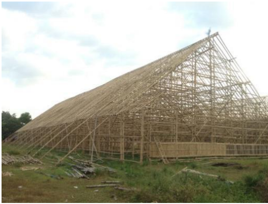
Figure 8. Warehouse bamboo frame
