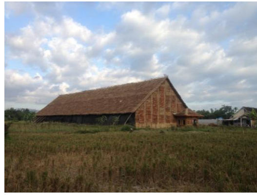
Figure 11. A ready Atag warehouse
