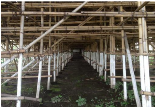
Figure 9. Warehouse floor and foundation
