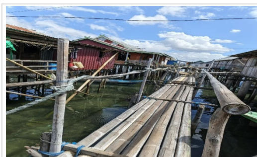
Figure 2. The use of ironwood ( kayu ulin , Eusiderodoxylon zwageri ) and bamboo as structural supports for stilt houses and interconnecting bridges in the original Roma Toloh construction of the Wuring settlement, East Nusa Tenggara
