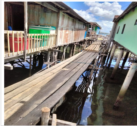
Figure 3. The shift in Roma Toloh construction systems post-1992 tsunami: the structure on the left retains the original wooden column construction, while the structure on the right utilizes a reinforced concrete column system
