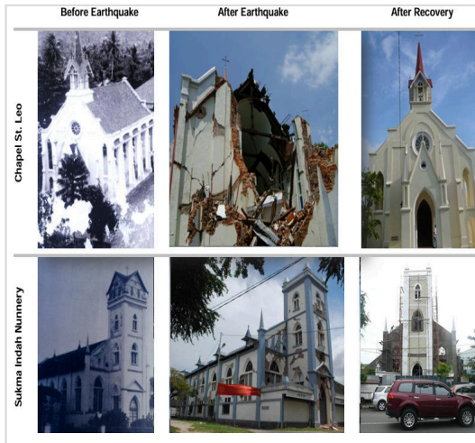
Figure 8. Catholic Monastery building conditions pre-post-earthquake and post recovery
