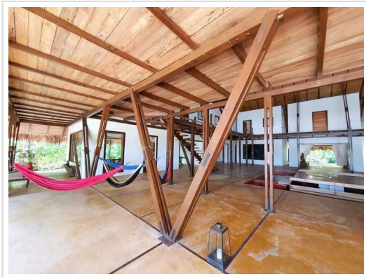
Figure 7. Wooden structural joint of the main resort building
