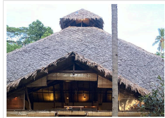
Figure 8. Roof form and materials of the main resort building
