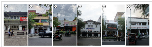
Figure 2. Building Exterior, (a) Jogja Library Center, (b) Nam Hien, (c) Sari Ilmu, (d) Kimia Farma, (e) Enteng, and (f) Sumber Husodo
