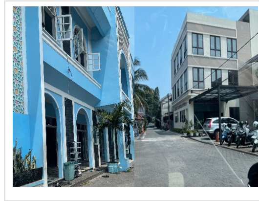
Figure 10. Mosque and Graha LDII building in Nurul Iman Mosque Complex LDII
