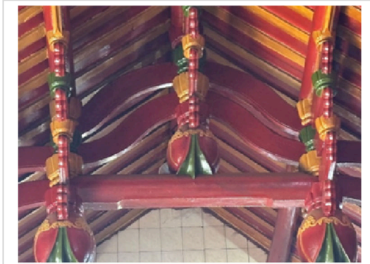
Figure 12. Chuan-Dou Construction in the truss of Rumah Rakit
