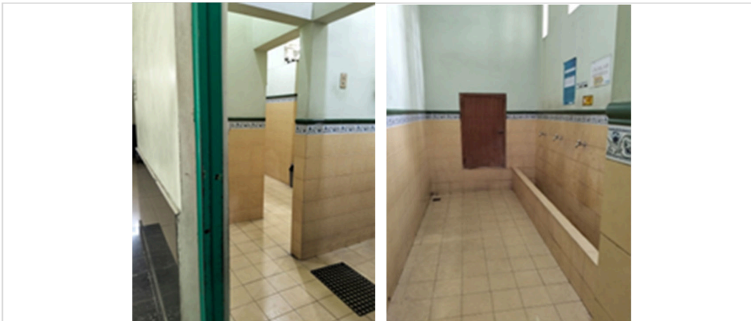
Figure 8. Women's ablution room 2 with a wall element design that makes the women who perform the ablution invisible from the outside
