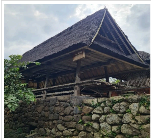
Figure 8. Typical view of foundation made from river stone
