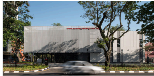
Figure 1 and 2. Shows the exterior view of Sunway Sales Gallery
