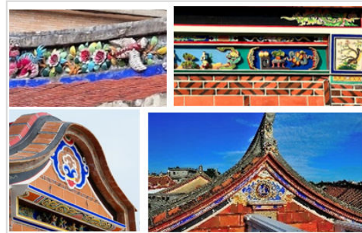
Figure 10. Chien Nien technique, a Fujian style colorful porcelain artwork on the facade, roof ridge, and gable Source: Online web: Huitu.com
