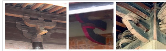
Figure 5. Simple wooden Dougong and stone Dougong as beams to support the extended roof Source: People's Government of Fujian Province, 2023
