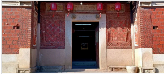
Figure 3. Red brick wall facade with white granite base Source: ICHE: International Conference on Humanities and Education 2022 (Ye and Tao 2022)
