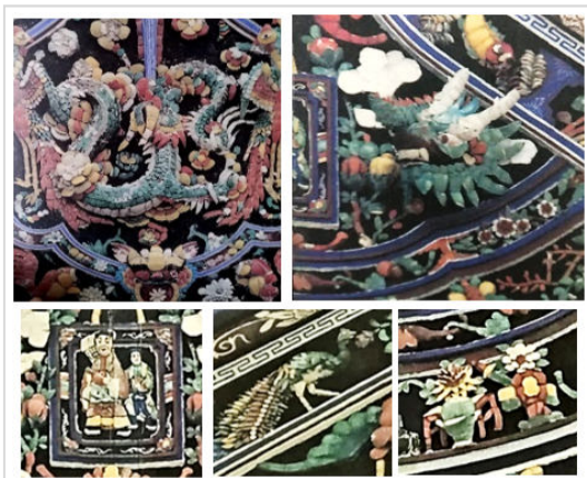
Figure 21. Closed-up of an external gable with Hokkien Chien Nien dragon, human figure, phoenix, and flora
