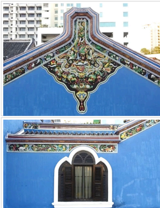
Figure 20. Ceramic shard decoration using the Hokkien Chien Nien technique on the gable facade Source: THE Vibes 2022, and taken by the author
