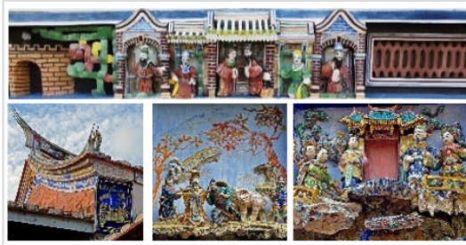
Figure 12. Painted Chai Hui on porcelain artwork on the building facade Source: online Web: Huitu.com
