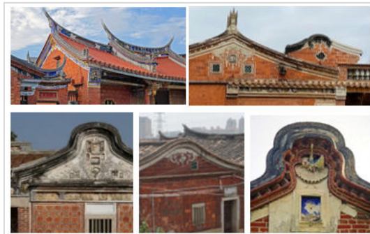
Figure 8. Swallowtail roof and horseback ridge gable roof (water and metal elements) can be found in most of the Southern Fujian architecture Source: People's Government of Fujian Province 2020
