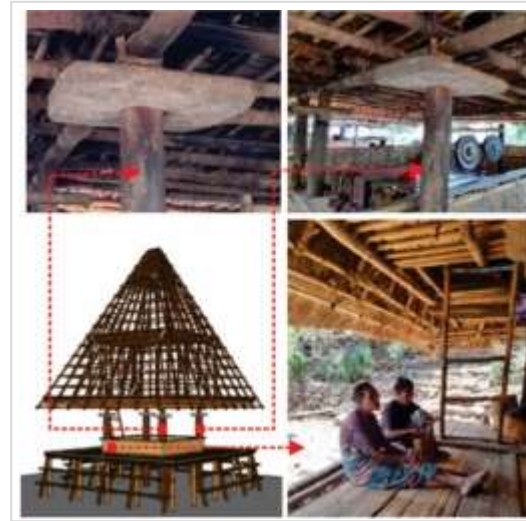
Figure 4. Fala house upper construction system
