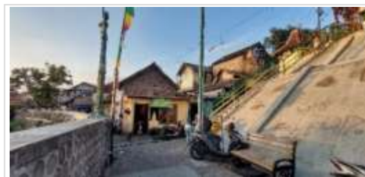
Figure 4. Bottom side of the Kali Code River embankment
