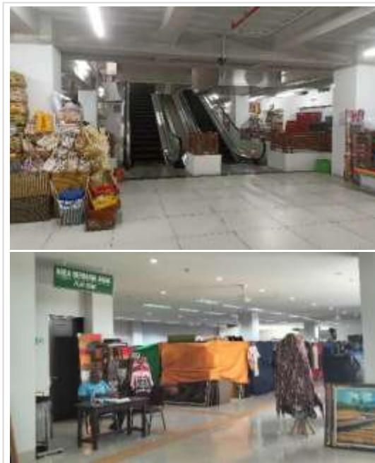
Figure 8. Description of the interior conditions of traditional market buildings undergoing modernization
