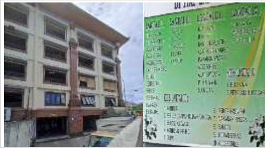
Figure 7. An overview of a multi-storey traditional market building is presented with the appearance of the building and signage indicating the type of space for each floor
