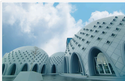
Figure 5. MAKT arch portal
