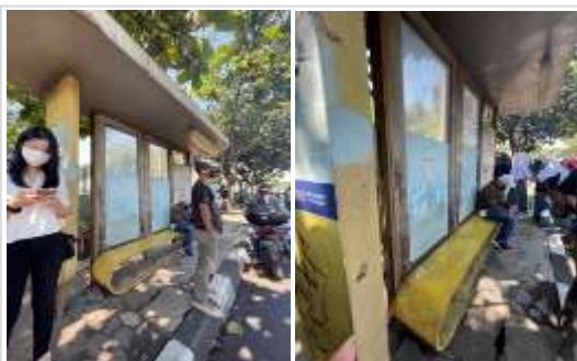
Figure 2. Documentation of survey of Soekarno Hatta bus stop, Bandung
