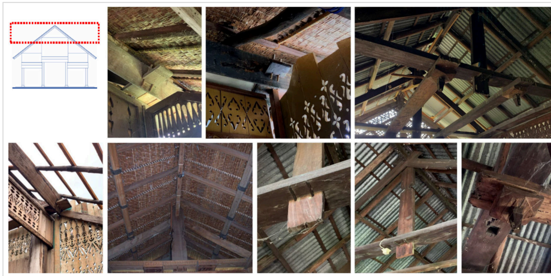
Figure 16. Roof frame construction documentation in Rumoh Aceh
