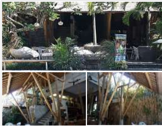
Figure 4. Building materials for this restaurant Above: Lower front terrace - frangipani trees, upper floor facing terrace. Bottom-left: Bamboo pole-roof frame, natural stone terrace walls, glass balustrade, glass-block walls, open alang-alang roof
