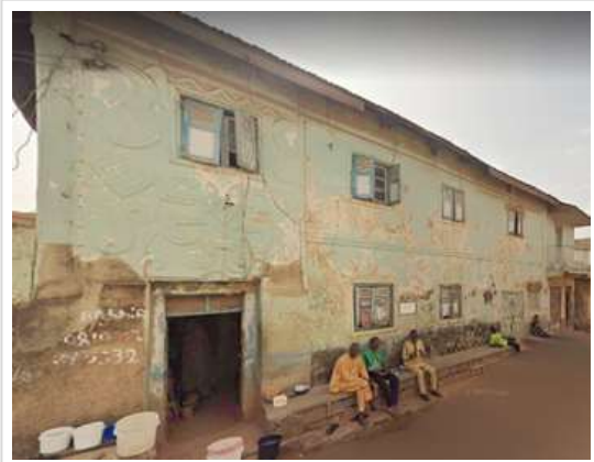
Plate 13. Picture of case study 8. Location: School Line Street, Jos
