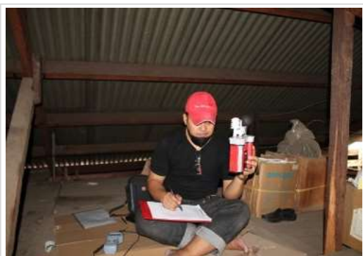
Figure 1. The attics were converted to a warehouse in the residential building in Cicadas, Bandung City
