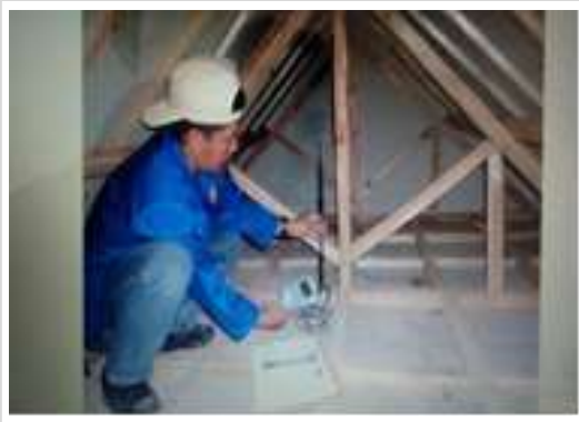
Figure 6. Measuring implementation of ambient temperature in the model room
