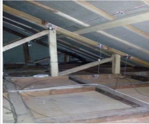
Figure 7. Installation and testing of Hi-Logger equipment
