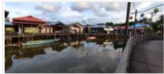
Figure 1. Ironwood as a building material in all houses
