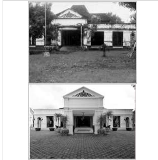
Figure 3. Dalem Wuryaningratan before being revitalized (left). The building after revitalization (right). Source: (Purnomo et al. 2022)
