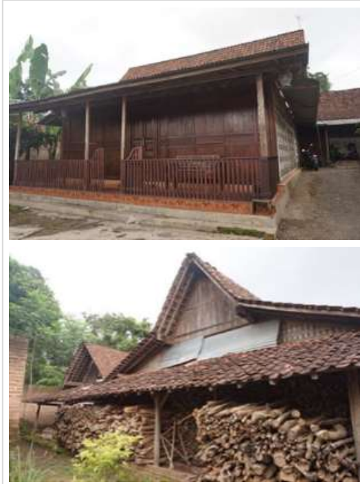
Figure 8. The photo shows the amper (left) and ampok (right) rooms in Osing house
