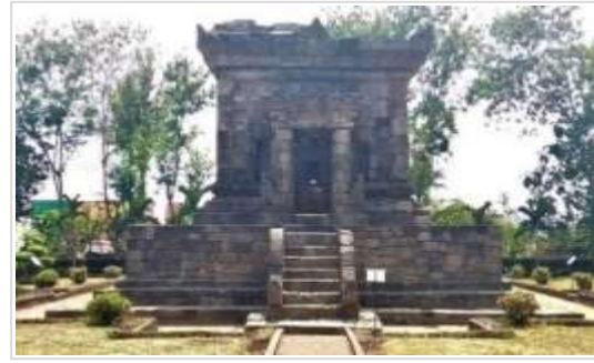
Figure 3. Existing photos of the current Badut Temple
