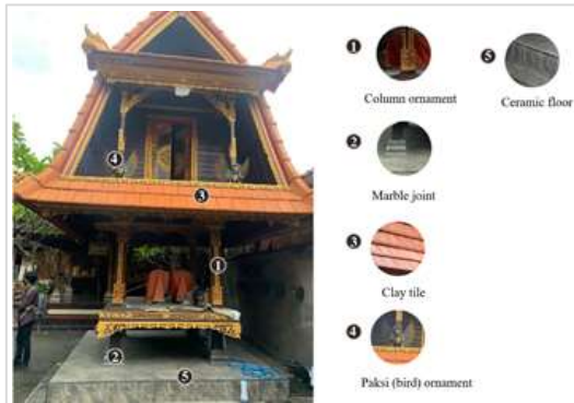
Figure 4. The shape of the Jineng (Barn) building which has undergone a transformation in form and function
