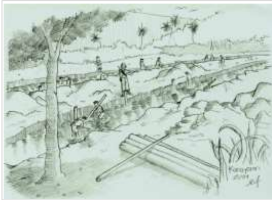
Figure 7. Traditional Banjar community canal-based road construction
