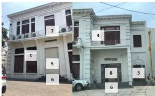
The latest texture of the main facade
