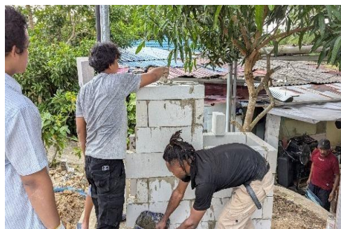
Figure 3. Construction Process and Final Installation of the Low-Smoke Incinerator
