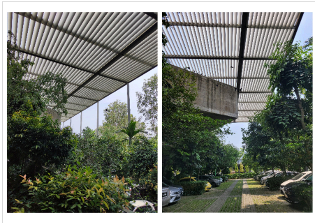
Figure 1. Slim Columns and Brise Soleil Louver Structure (left)
